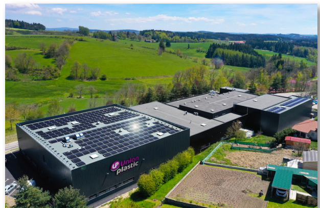
The solar panels at the UPP Union Plastic site in St Didier en Velay.
